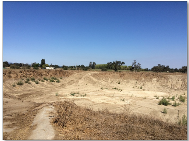
Manure Pond Before Paving (Sept 2015)
