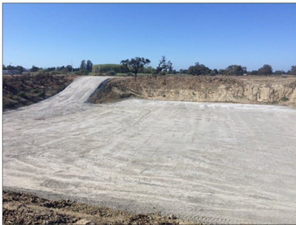
Manure Pond After Paving (Sept 2015)
