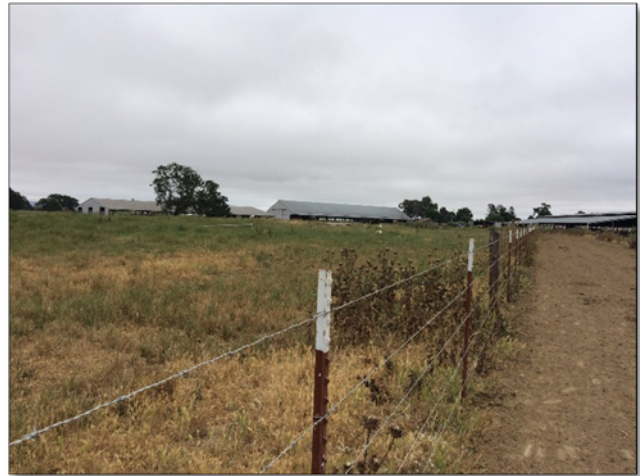
Clean water culvert at inlet and vegetated buffer managed by flash grazing (June 2016).
